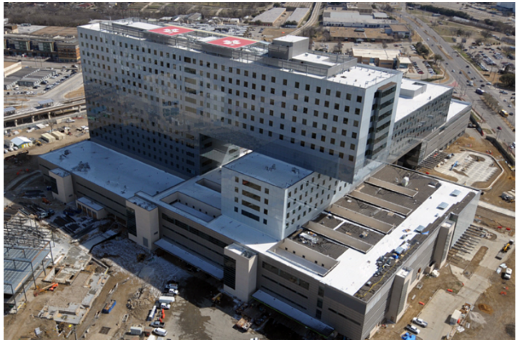
Parkland Hospital under construction
